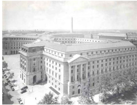
Post Office Department Headquarters, Washington, D.C., July 19, 1934
