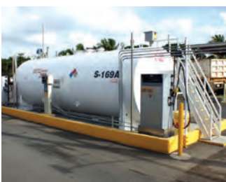
NAVAUDSVC reviewed Craney Island bulk fuel storage facilities.
