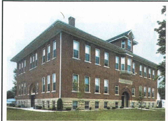
Camden Commons, in Preble County, Ohio, is an old schoolhouse rehabilitated into 14 units of housing for the elderly. Camden Commons was a LIHTC investment project of Ohio Capital Corporation, a member of National Association of State and Local Equity Funds.
