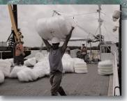
Unlike hard boom, sorbent boom does not have an attached skirt. Once saturated with oil, sorbent boom must be removed and properly disposed of. It is used to both contain and absorb oil on the water surface.
