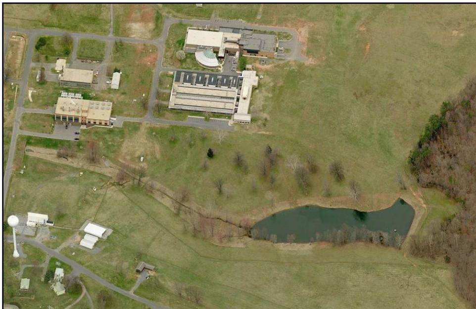
Figure 3-8. Aerial Photograph of Intermittent Stream and NIHAC Reservoir (Looking North)
