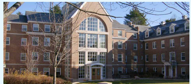
First ENERGY STAR labeled dormitory: Congreve Hall, University of New Hampshire, Durham, NH
