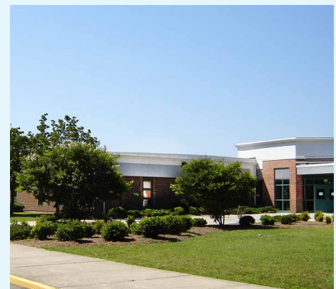
Bruton High School's geothermal system is helping to keep energy costs low.
