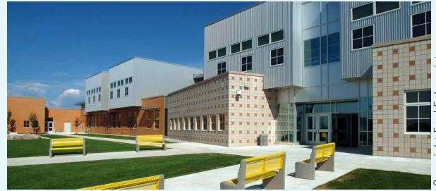
First ENERGY STAR labeled building that had also achieved "Designed to Earn the ENERGY STAR" for its design plans: Kinard Junior High School, Fort Collins, CO
