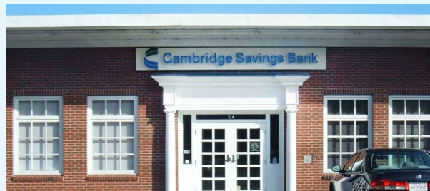
Smallest ENERGY STAR building: Cambridge Savings Bank's Burlington Banking Center, Burlington, MA. At 2,313-square-feet, it is about the size of the average American home.
