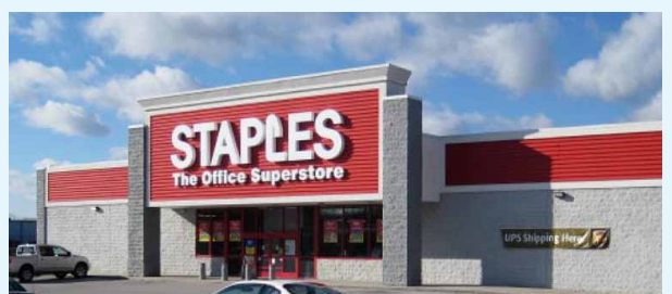
First ENERGY STAR labeled office supply store: Staples, Crossville, TN
