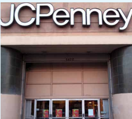
Built in 1928, JCPenney's Huntington Park store benefitted from a long-standing corporate commitment to energy efficiency.
