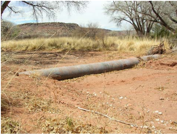
c. Flume 2, pipe laying on surface of arroyo
