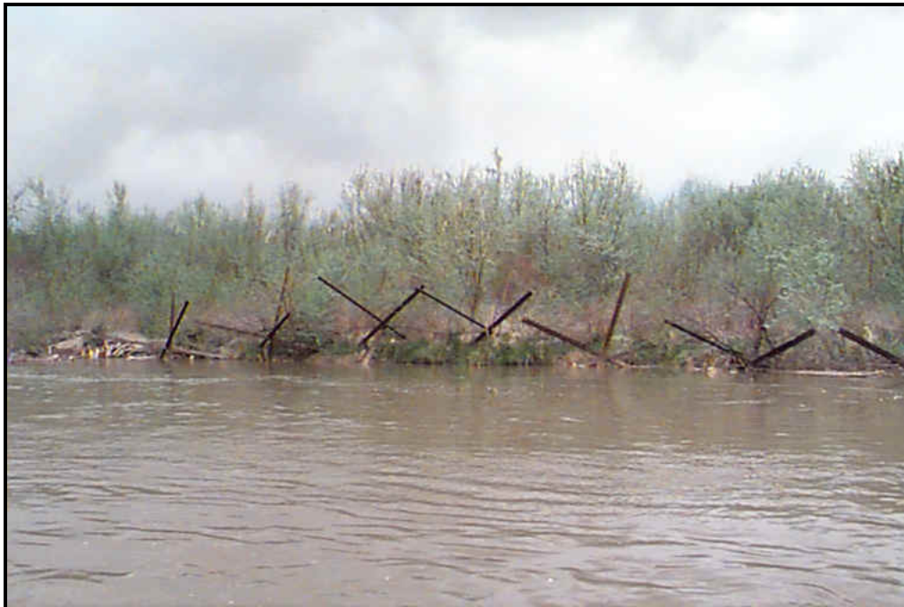
Figure 27. Jetty jacks lined along the bank of the Rio Grande trap sediment and plant material during flooding events, stabilized over-bank areas over the course of several years.
