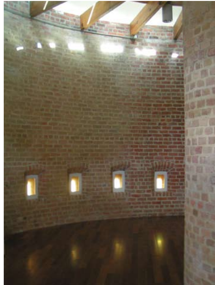
Historic battlement towers on Jackson Barracks were carefully restored after sustaining significant damage and now serve as ‘VIP’ quarters.
