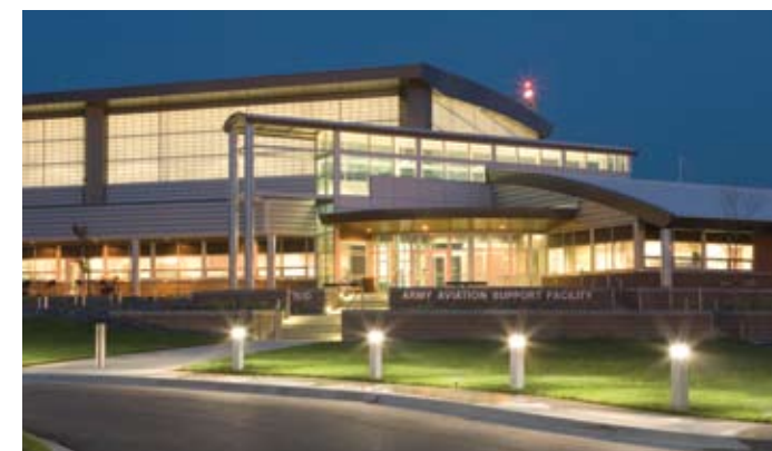
Forty-eight skylights provide the facility with daylight, and just underneath the roof, a 620-foot light shelf reflects low-angle winter light deep into the structure.
