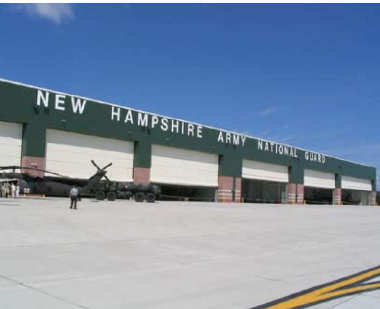
New Hampshire Army National Guard’s Army Aviation Support Facility was completed in 2004 at an approximate cost of $21 million.
