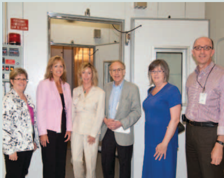
Inspecting the New Freezer: (from left) Kathleen Groover, of Fisher BioServices, with Marianne Henderson, Karen Pitt, Joseph Fraumeni, Shelia Zahm, and Mark Cosentino, repository contracting officer’s technical representative for SAIC-Frederick, Inc. (Photograph credit: Jonathan Summers)
