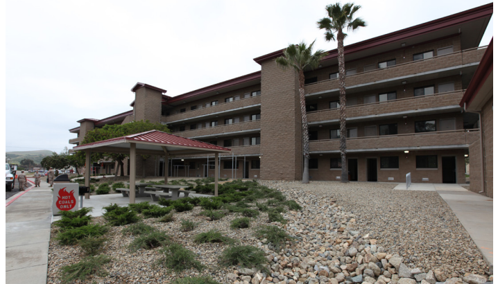
Apartment complex at Marine Corps Base Camp Pendleton, California. (Photo courtesy of Department of Defense.)
