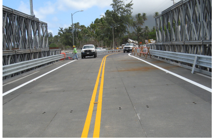
The new bridge almost ready for traffic.
