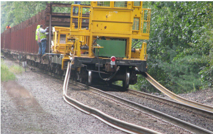
New double track for Haverhill Line.
