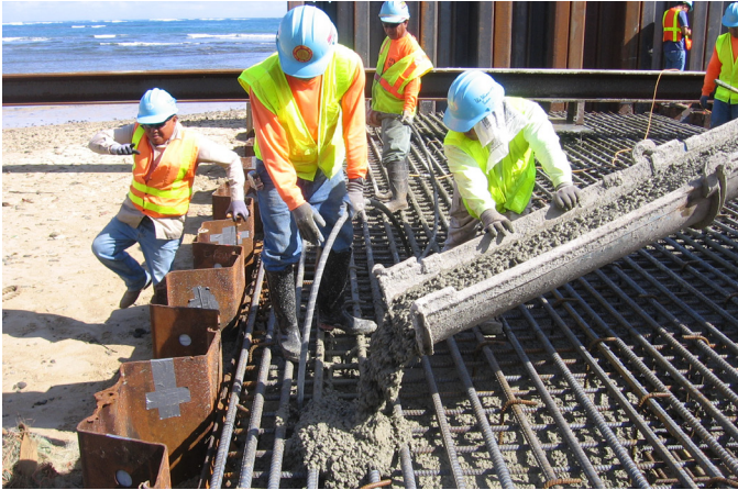
Pouring concrete for section of new bridge.
