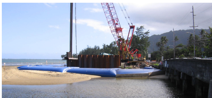
Preparing renovation of 84-year-old bridge, at right.
