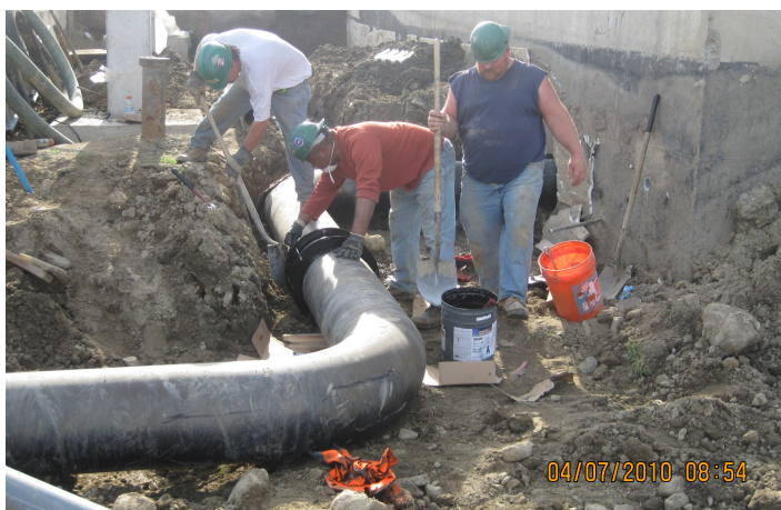
In Middletown, NY, the wastewater facility is being expanded, and new drainage pipes installed.
