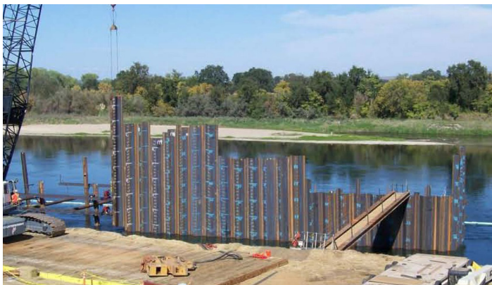
Installing coffer dam sheet piling for fish screen.
