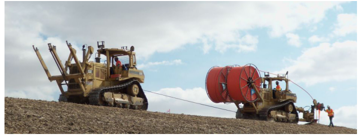
Laying cable to bring high speed Internet connectivity to rural areas.
