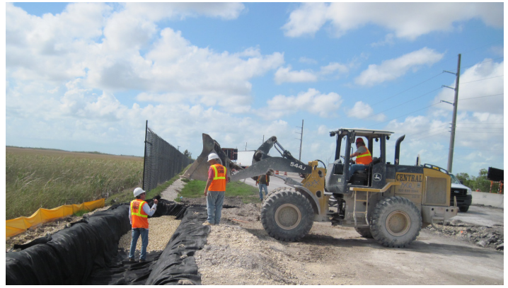
Redoing Florida highway includes new drainage as well as road widening.
