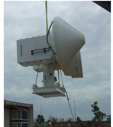
Final assembly of precipitation radar antenna.
