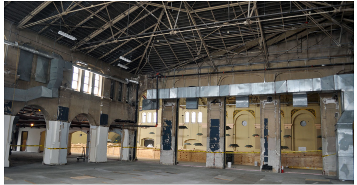
Repairs and renovations for the Smithsonian Institution.
