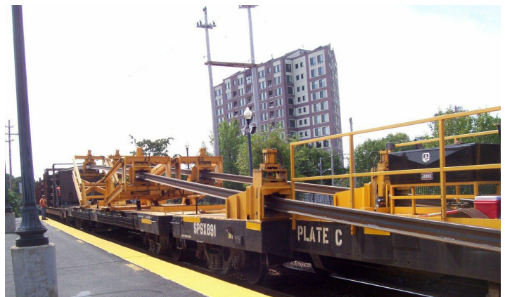
Transporting new double track.
