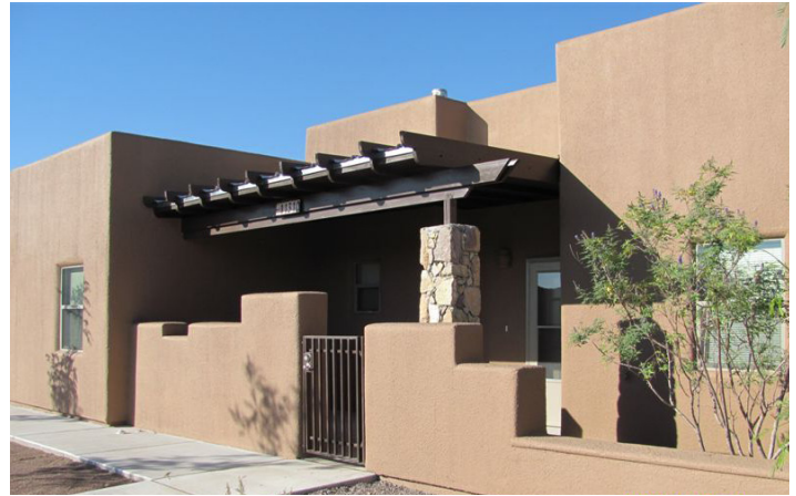
One of the new homes for the Pueblo Nation in El Paso, TX.
