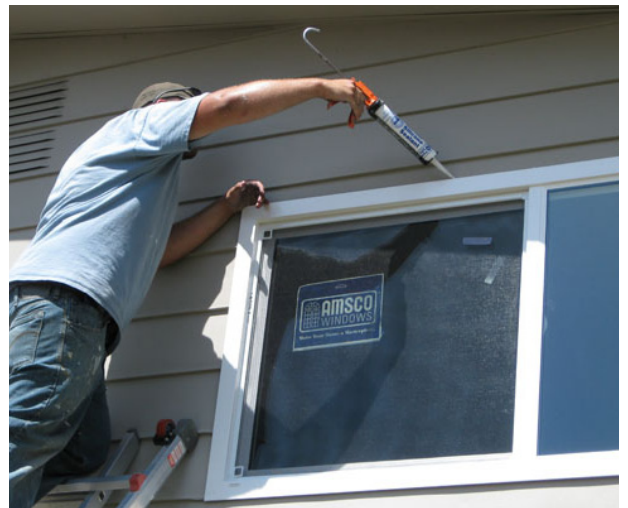
Worker seals new energy-efficient window on an Ohio home.
