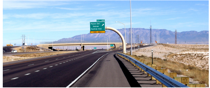
In June 2010, the New Mexico Department of Transportation completed work on I-40, the first major Recovery Act transportation project in the state.
