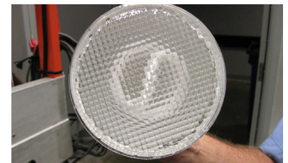
Replacing incandescent floodlights with efficient compact fluorescent models at the Virginia Beach Convention Center.
