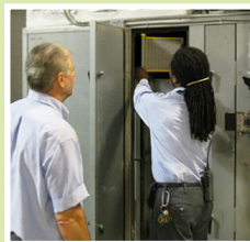
Installing new MERV 14 HVAC filters at Virginia Beach Convention Center
