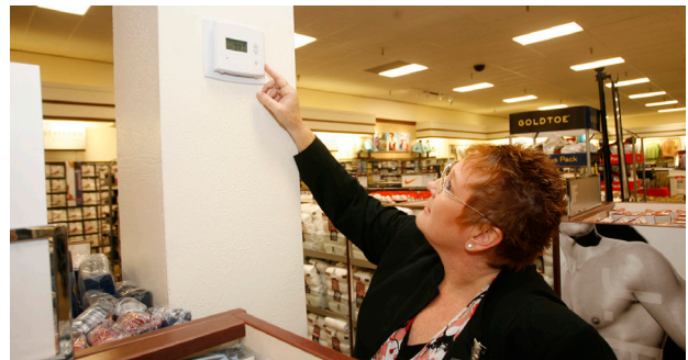
JCPenney's store manager, Nancy Gutzmer, is programming her lights to come on at store opening and to shut off at store close. The unit has the ability to program general lighting and accent lighting
