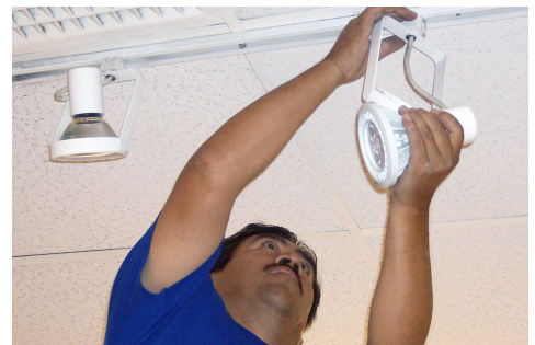
Replacing old lighting with light emitting diodes (LED) at JCPenney.
