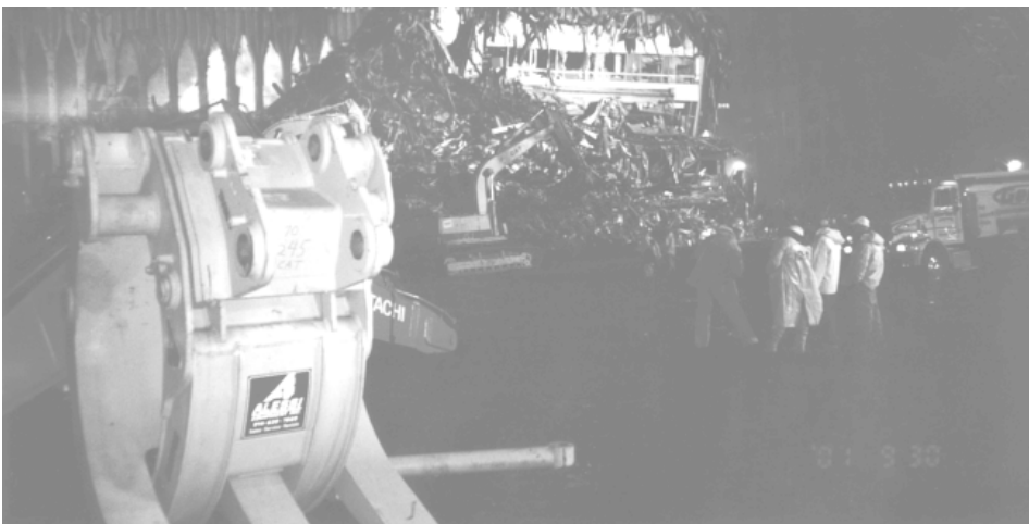
This is a photo of a grappler hook; an example of the kind of equipment used by the ironworkers to remove massive pieces of twisted metal. The skeleton of a WTC tower is in the background.
