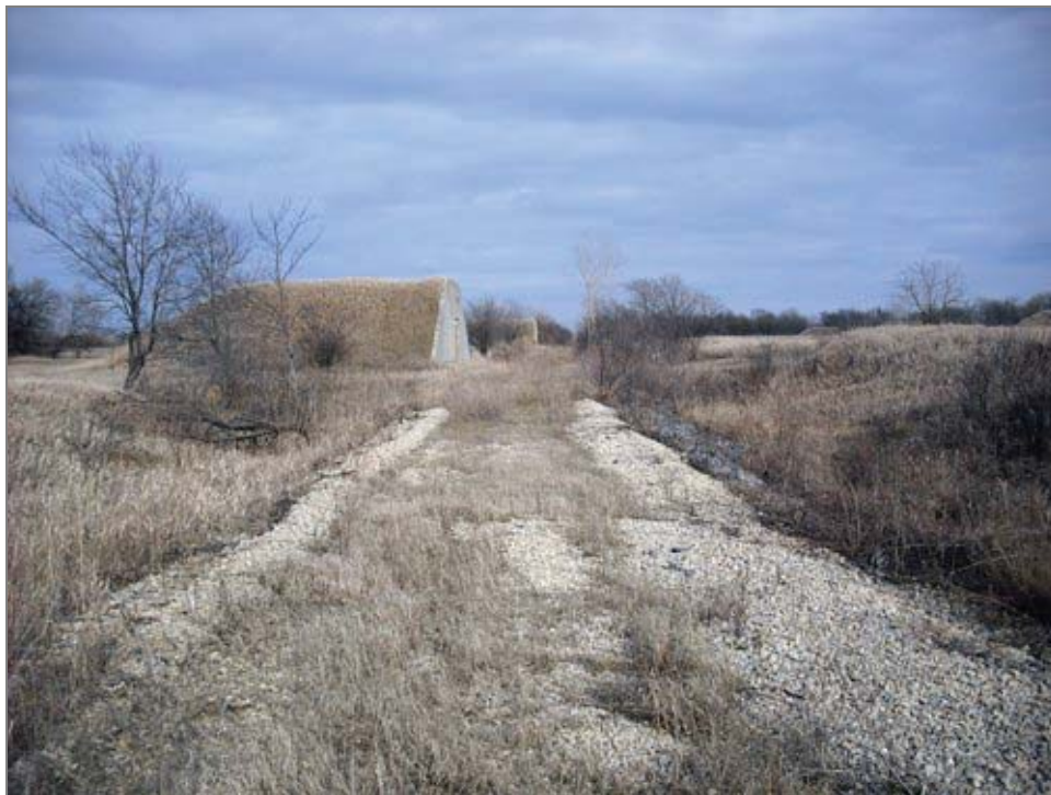
FIGURE 13. INERT STORAGE WAREHOUSE AREA GROUP 63 IGLOOS AND ABANDONED RAILROAD SIDING, FACING EAST
