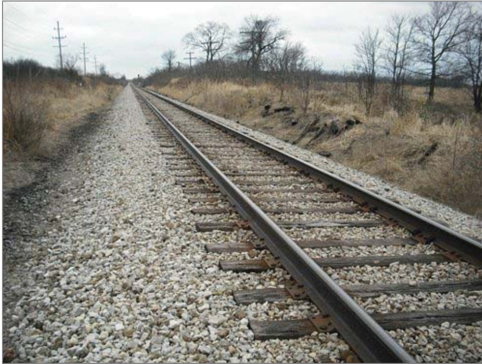
FIGURE 7. C&M / C&A / UP RAILROAD, FACING SOUTHWEST
