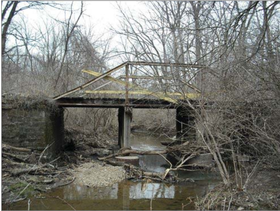
FIGURE 11. GRANT CREEK BRIDGE, FACING WEST
