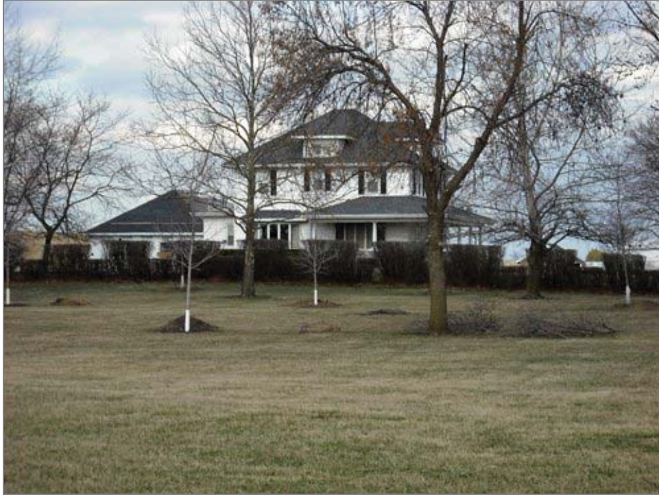
FIGURE 9. 26953 STATE ROUTE 53, HOUSE, FACING NORTHEAST
