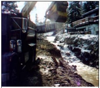
Shown above, sediment removal and rechannelization work along the South Fork Squaw Creek. Note the original elevation of debris on the right side of the creek. Shown below, the creek after emergency work to divert water flow back to the existing channel. The debris piled up to the top of the deck rail on the left, about 8 feet above the top bank of the creek.
