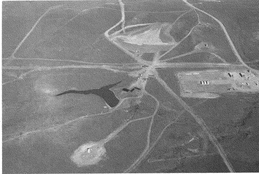
Coalbed Methane roads, drill pads, compressor station and reservoir for discharge water
