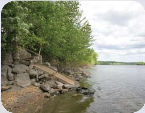
Combined sewer overflow (CSO) discharges directly into the Connecticut River.
