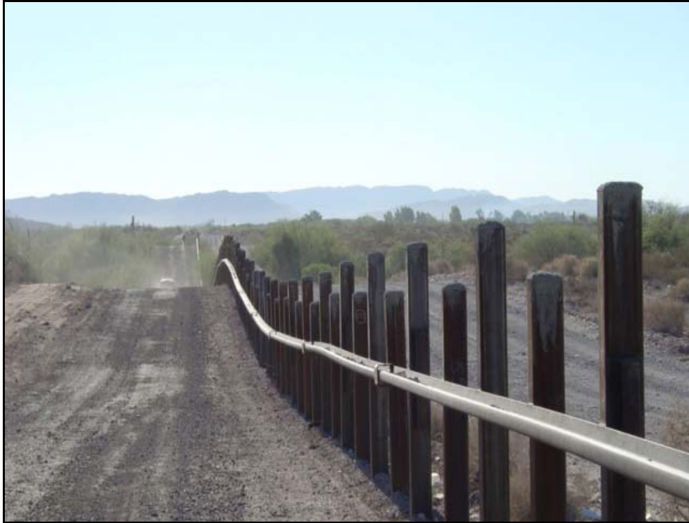
Figure 1-2. Post-on-Rail-Style Vehicle Fence (Fence Type VF-1)
