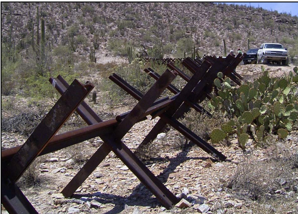
Figure B-2. Normandy-Style Vehicle (Fence Type VF-2)
