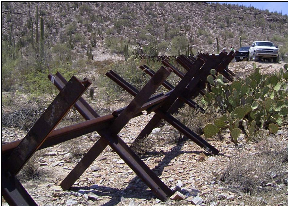
Figure 1-3. Normandy-Style Vehicle Fence (Fence Type VF-2)
