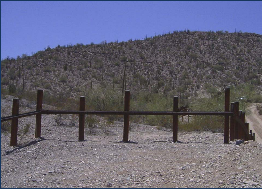
Figure 2-1. Photograph of Post-on-Rail Fence
