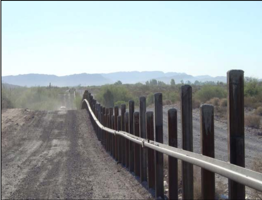
Figure B-1. Post-and-Rail Vehicle Fence (VF-1)
