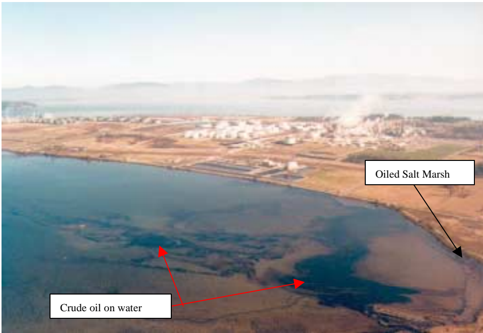
Figure 4. Oil slick in southern Fidalgo Bay on February 22, 1991. March Point and the Texaco Oil Refinery can be seen in the background. Dark patches and streamers of crude oil are visible throughout much of the southern portion of the bay. Salt marshes and intertidal beaches were heavily oiled in this part of the bay (lower right portion of the photo).
