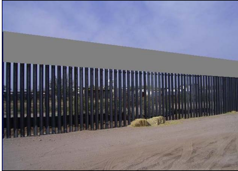
Figure 1-4. Personnel-Vehicle Fence Type-1 (PV-1)
