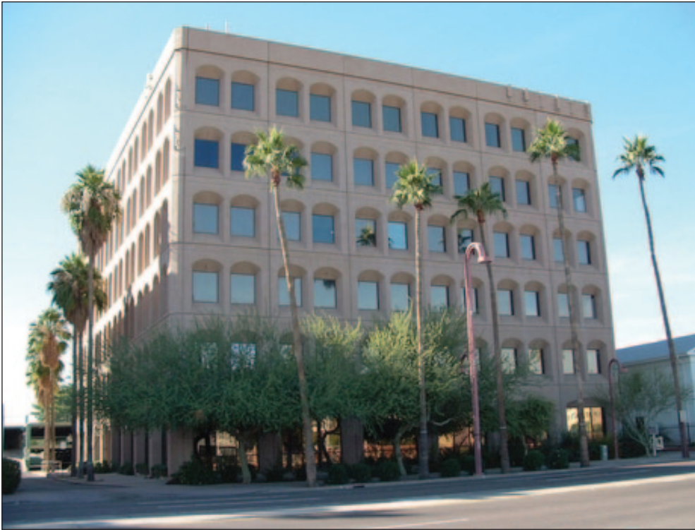
Arizona MultiBank CDC
