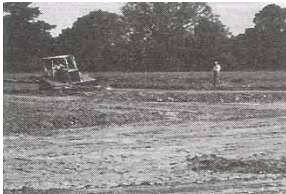
Grading the site: The first step in constructing a wetland.
