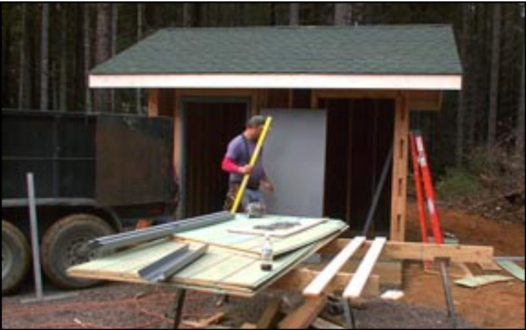
Figure 42: Old Sherwood Valley Rancheria pumphouse and treatment building construction, California.
