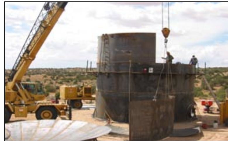
Figure 41: Construction of a 88,000 gallon water tank in White Mesa, Arizona.
