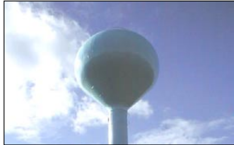
Figure 34: Completed 250,000 gallon elevated waste tower.
