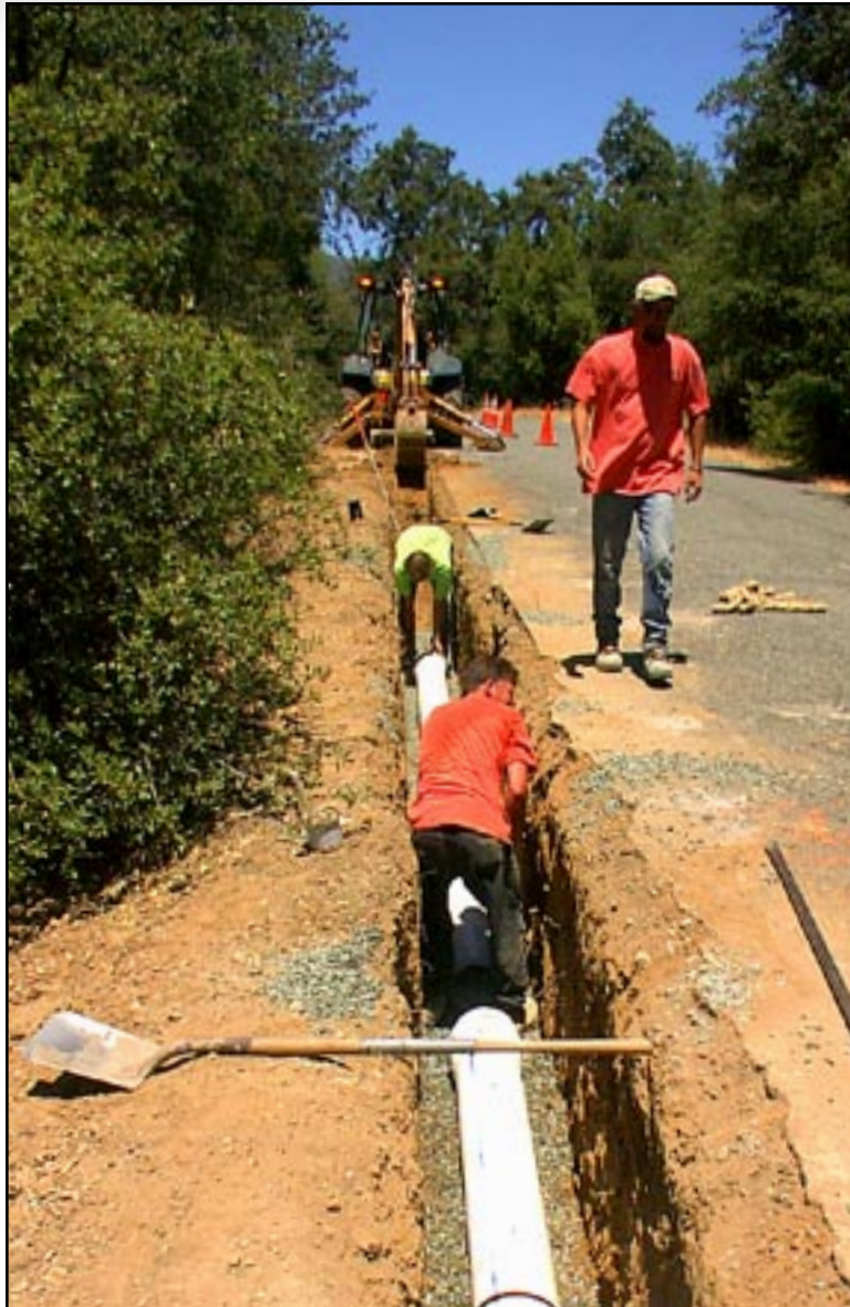
Figure 7: 8-inch PVC water main installation at Upper Lake Rancheria, California.
