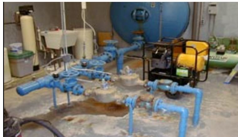
Figure 31: Interior piping of the Lac du Flambeau pumphouse
