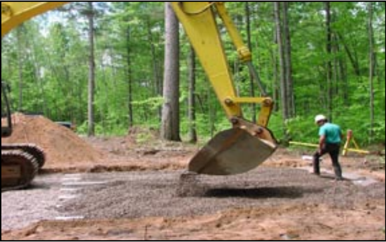
Figure 27: Construction of the drainfield for the sand filter treatment system.
