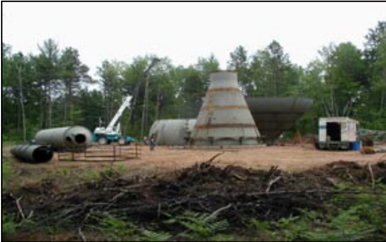
Figure 33: Construction of the 250,000 gallon water tower.
