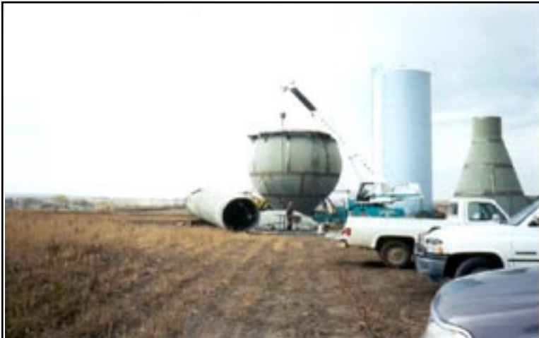
Figure 19: Erecting the middle section of the sphere.
