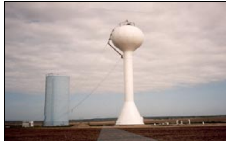
Figure 21: Completed water sphere; old tank will be abandoned.
