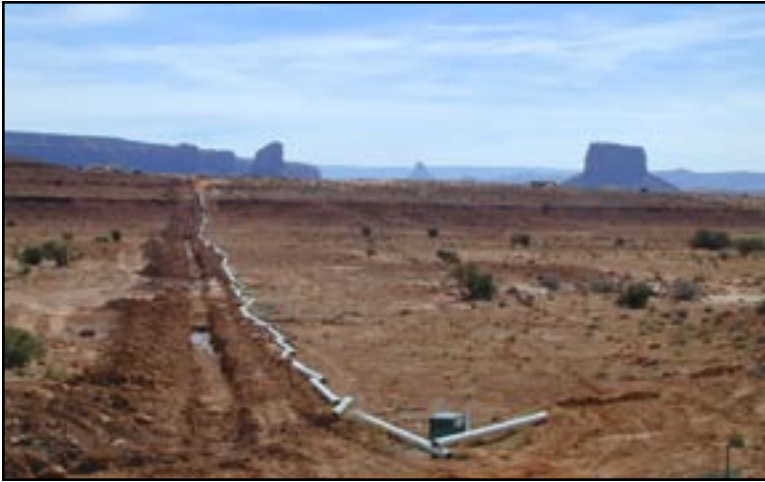
Figure 47: Waterline construction in Monument Valley, Arizona.
