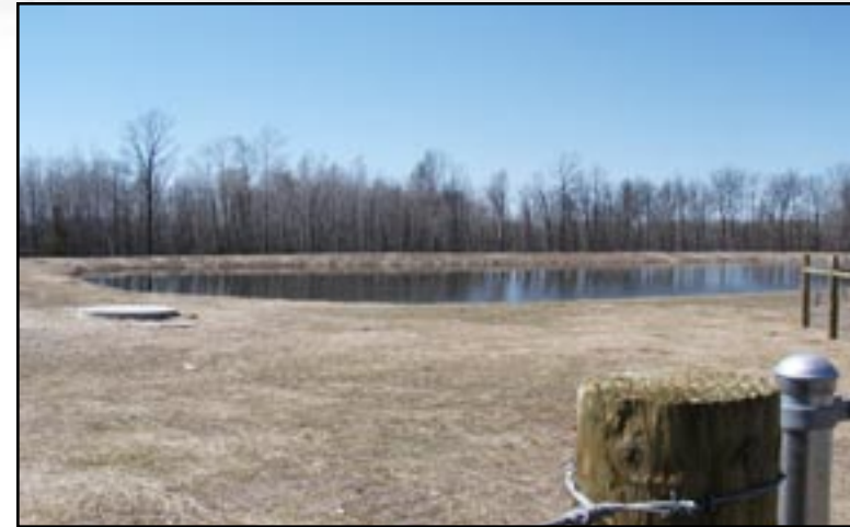
Figure 16: New primary cell in East Lake, Minnesota.
