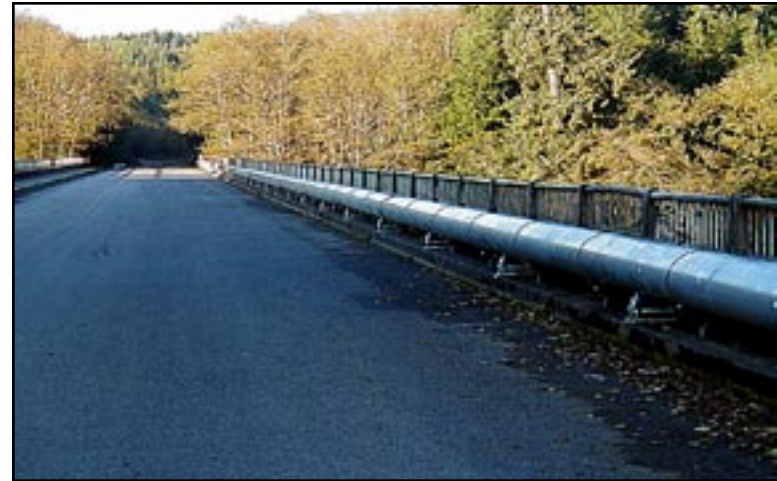
Figure 10: 18" steel casing on rollers with expansion joints crossing the Quinault River.
