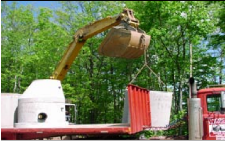
Figure 29: Unloading Manholes for sewer extension.
