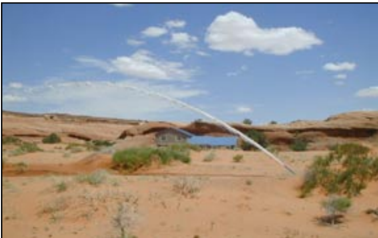
Figure 40: Flushing new water service line in Cane Valley, Navajo Nation.
