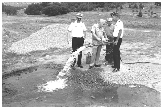
Figure 3-8. Test pumping a new well.
