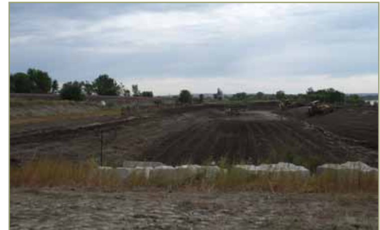
Reconstruction of the embankment.
