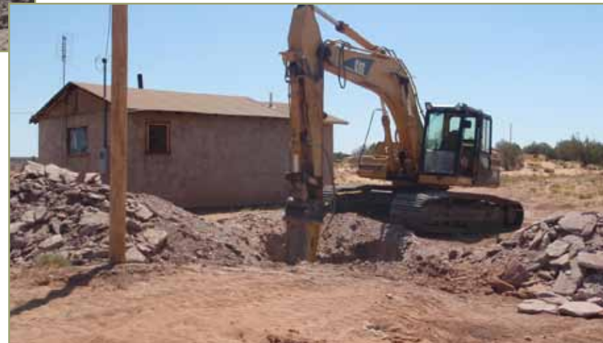
Installation of a septic tank drainfield system. 1
