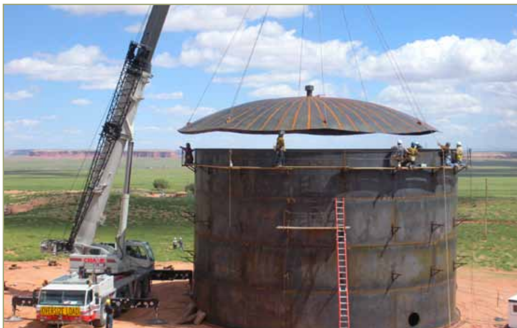
Steel water tank construction, Sweetwater, Arizona.
