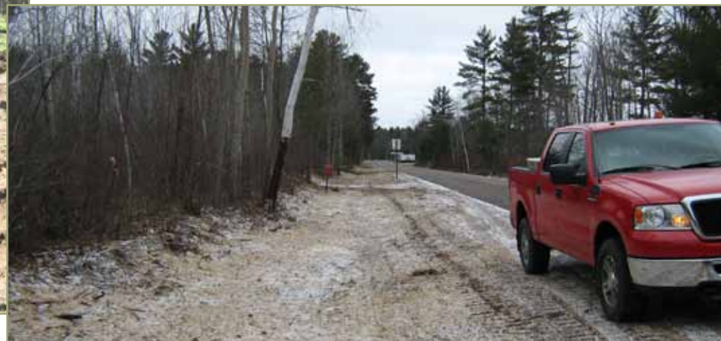
Right of way for the waterline.
