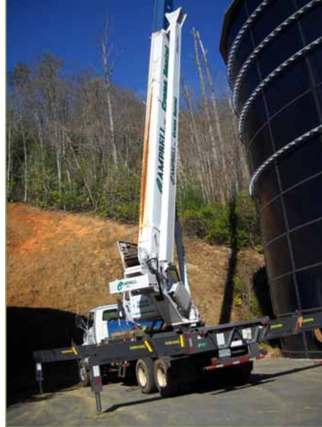
Erection of the water storage tank.
