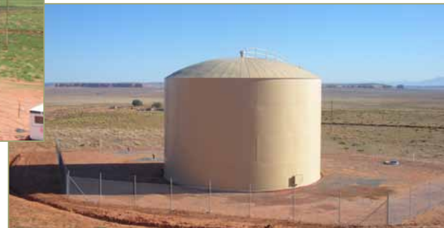
Completed 500k water tank construction, Sweetwater, Arizona.
