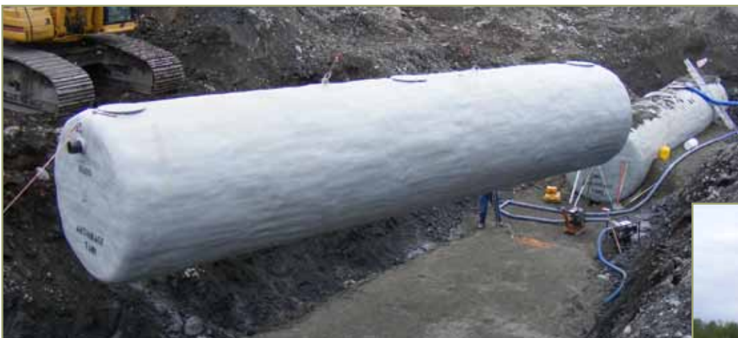
Placement of septic tanks.
