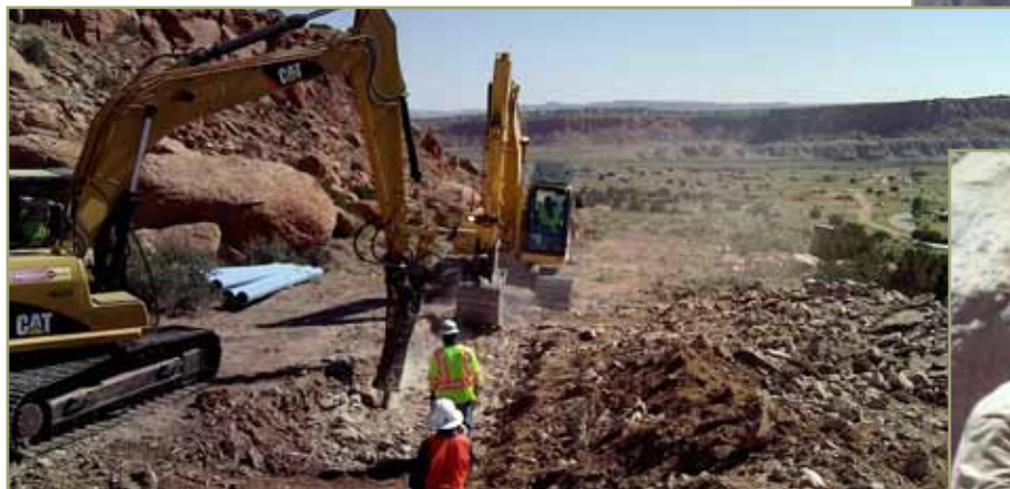
Clearing the right of way and rock excavation for the tank.
