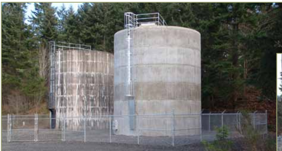
Completed and existing water storage tank.
