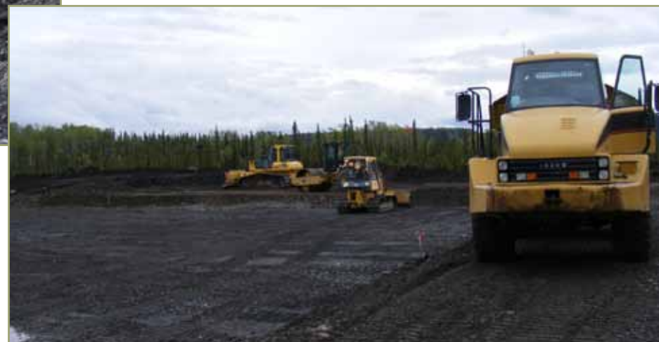
Construction to complete the lagoon.
