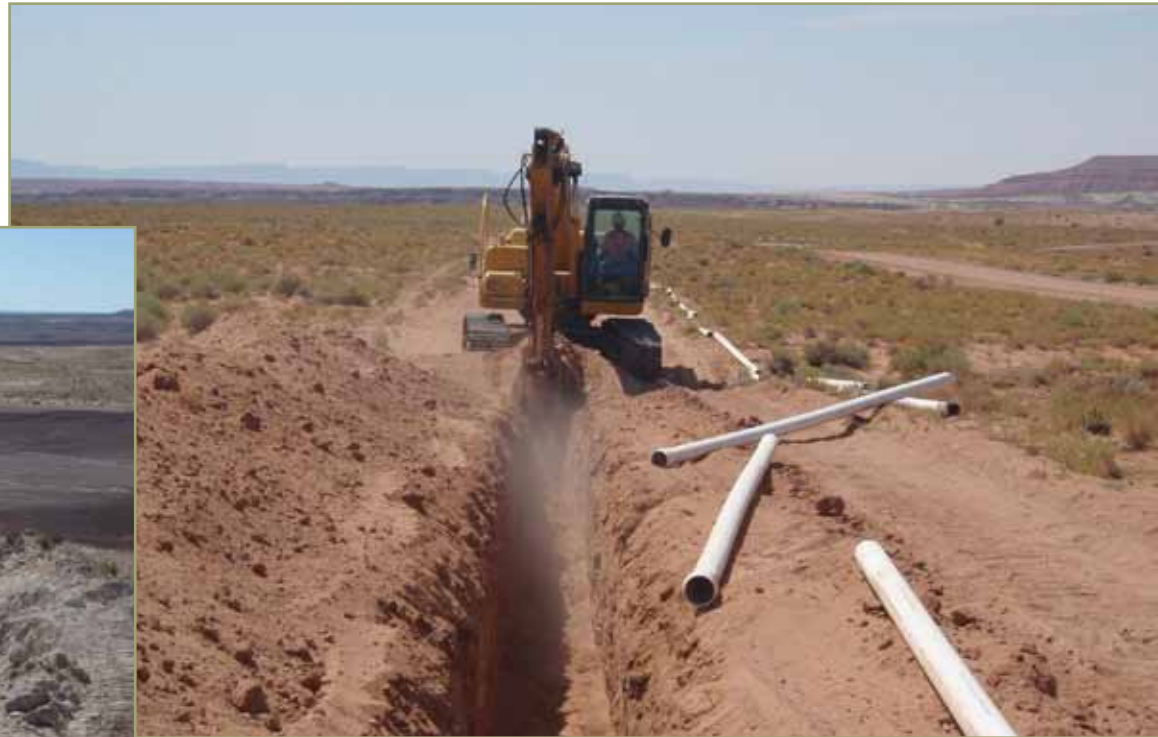
Construction of the waterline trench.
