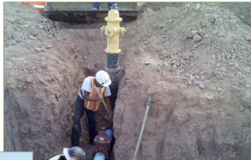
Construction of the water distribution line.
