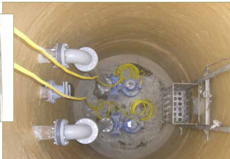
Renovated lift system.
