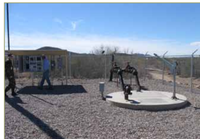
Completed sewage lift station.
