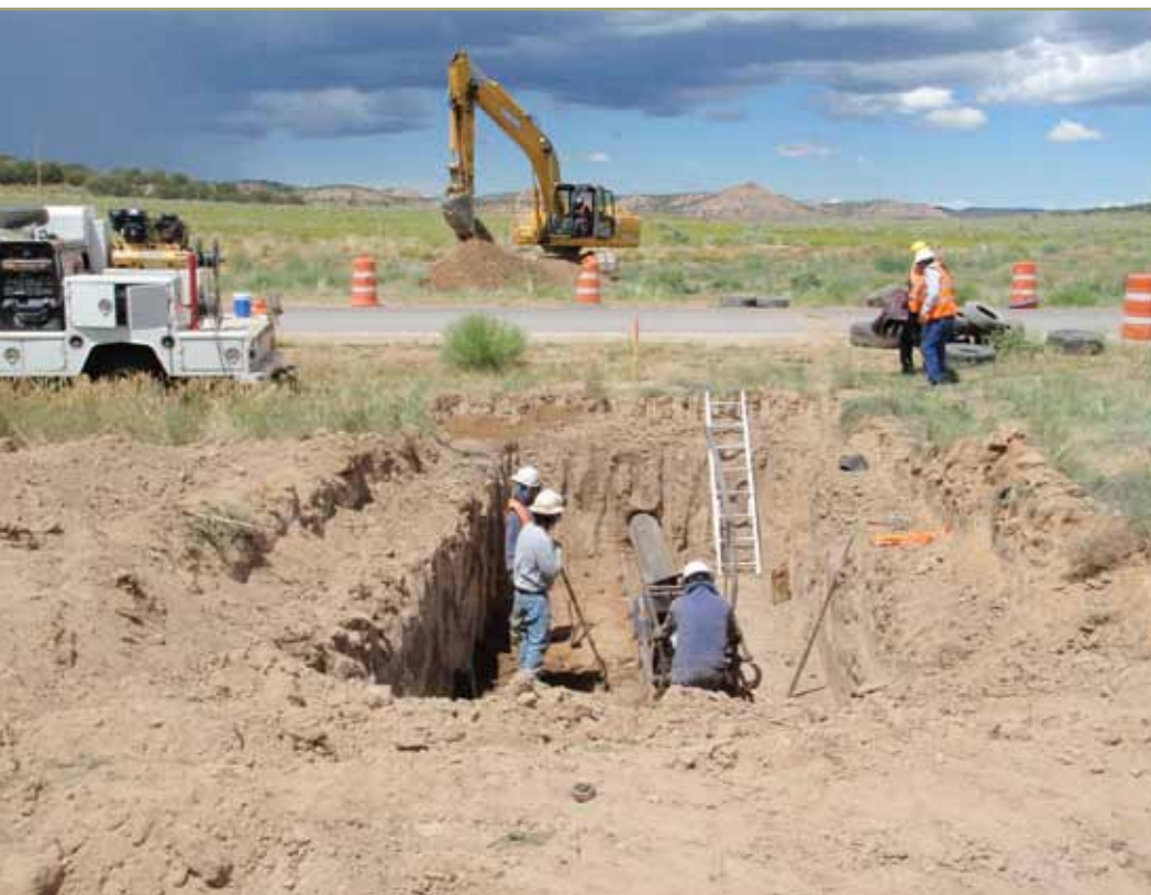
Directional road boring for waterline in Rock Point, Arizona.
