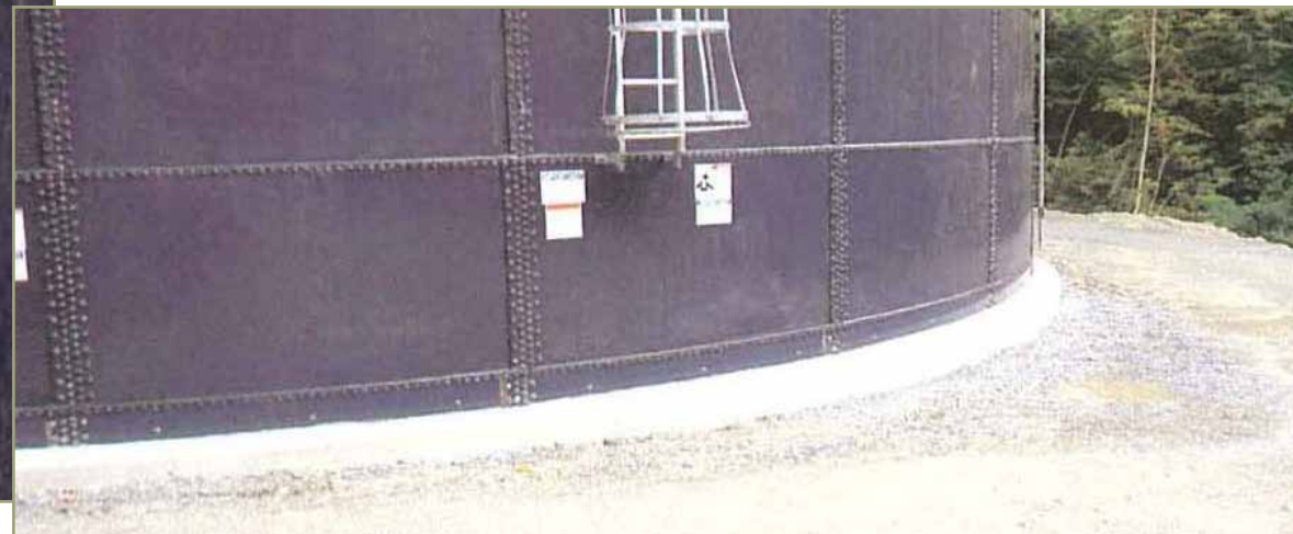
The reconstructed tank and foundation.
