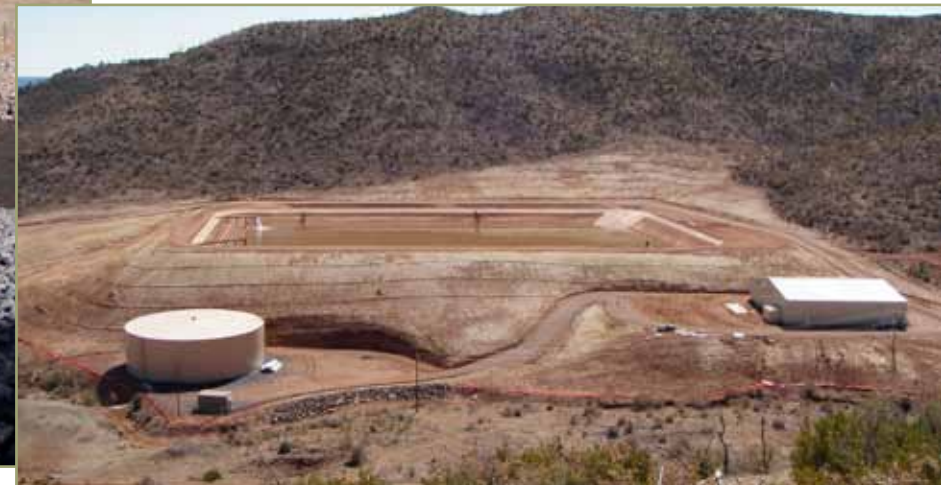
Overall of the completed water treatment plant.
