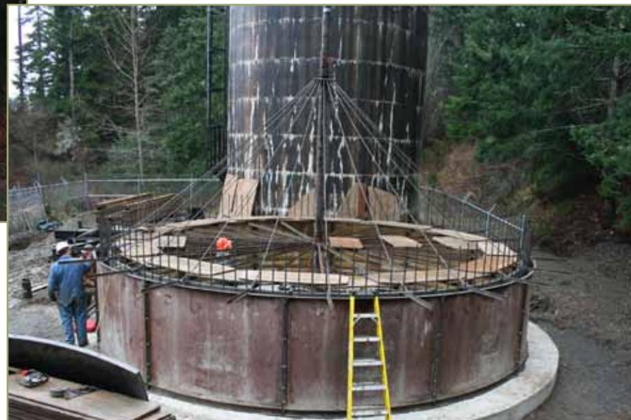
Construction of the concrete tank.
