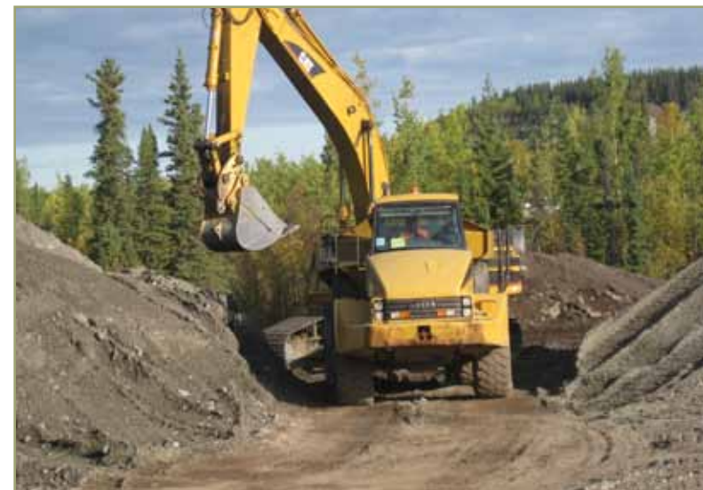
Removal of soil to complete the lagoon.
