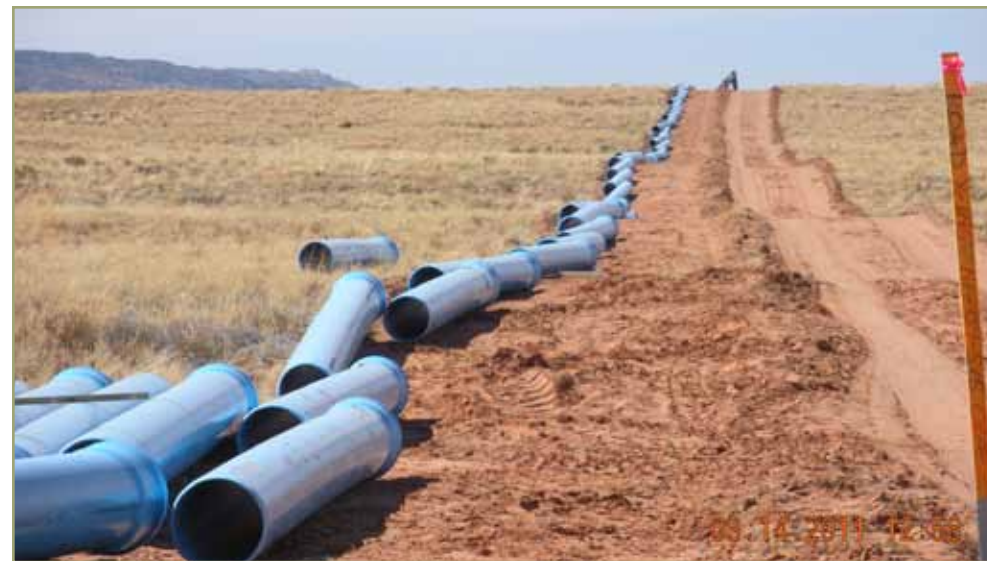
14" water distribution line construction in Sweetwater and Red Mesa, Arizona.
