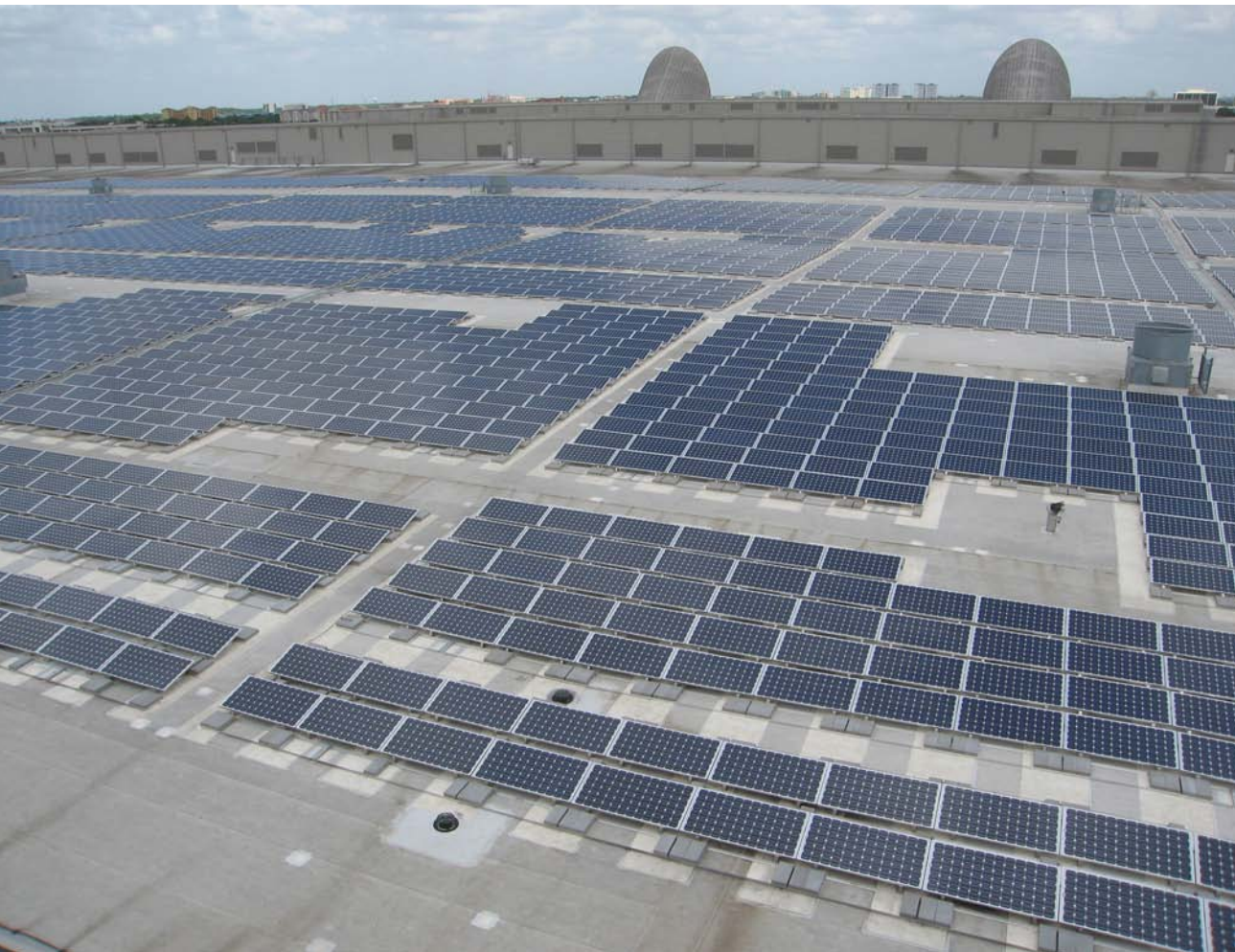
The solar array rooftop system on the South Concourse of the Orange County Convention Center in Orlando, Florida, was completed last year as a DOE Solar America Showcase. (Orange County Convention Center/PIX18077)
