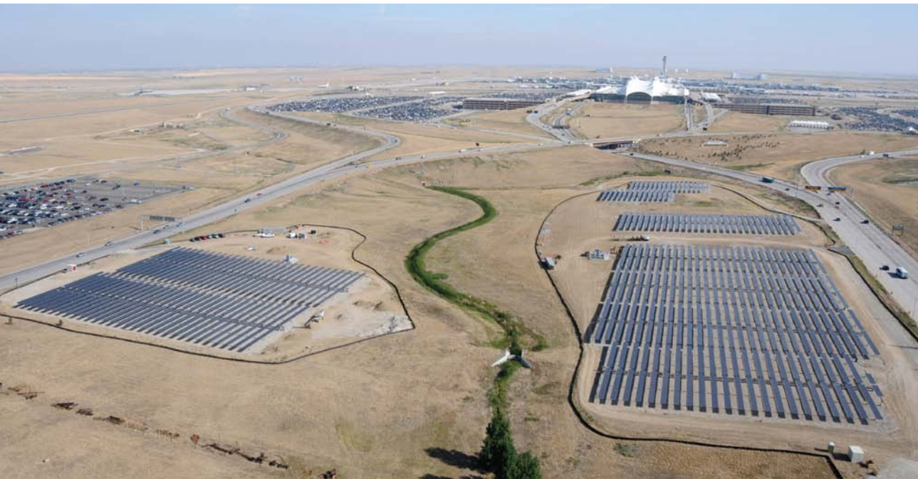
The Denver International Airport (DIA) features a 2 MW PV system. DIA is now host to a second 1.6 MW array system. (Denver International Airport/PIX18043)
