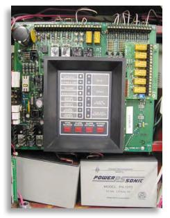
This fire alarm control unit (panel) includes two batteries to provide a secondary power supply.
