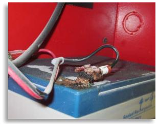
Regular visual inspections of fire protection systems should identify and correct problems like this corrosion on the battery terminal.
