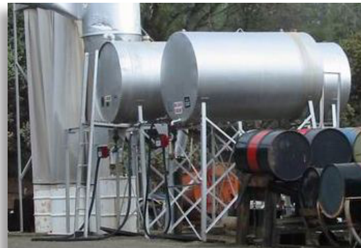
The wetted area of these horizontal storage tanks is based on a percentage of the tanks' surface area. (See Coffee Break Training 2006-18 for a discussion of steel tank supports.)
