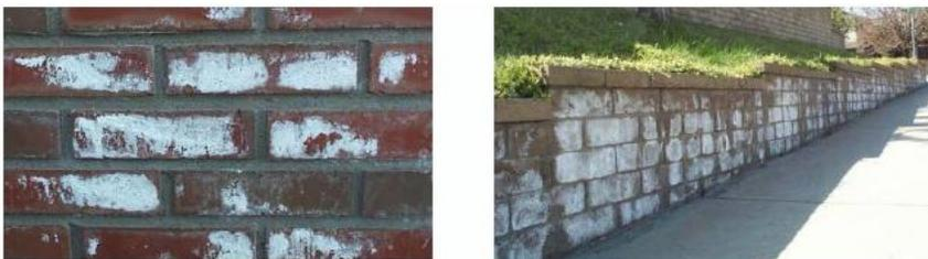
Figure 1. Typical white efflorescent salts on brick and block masonry
