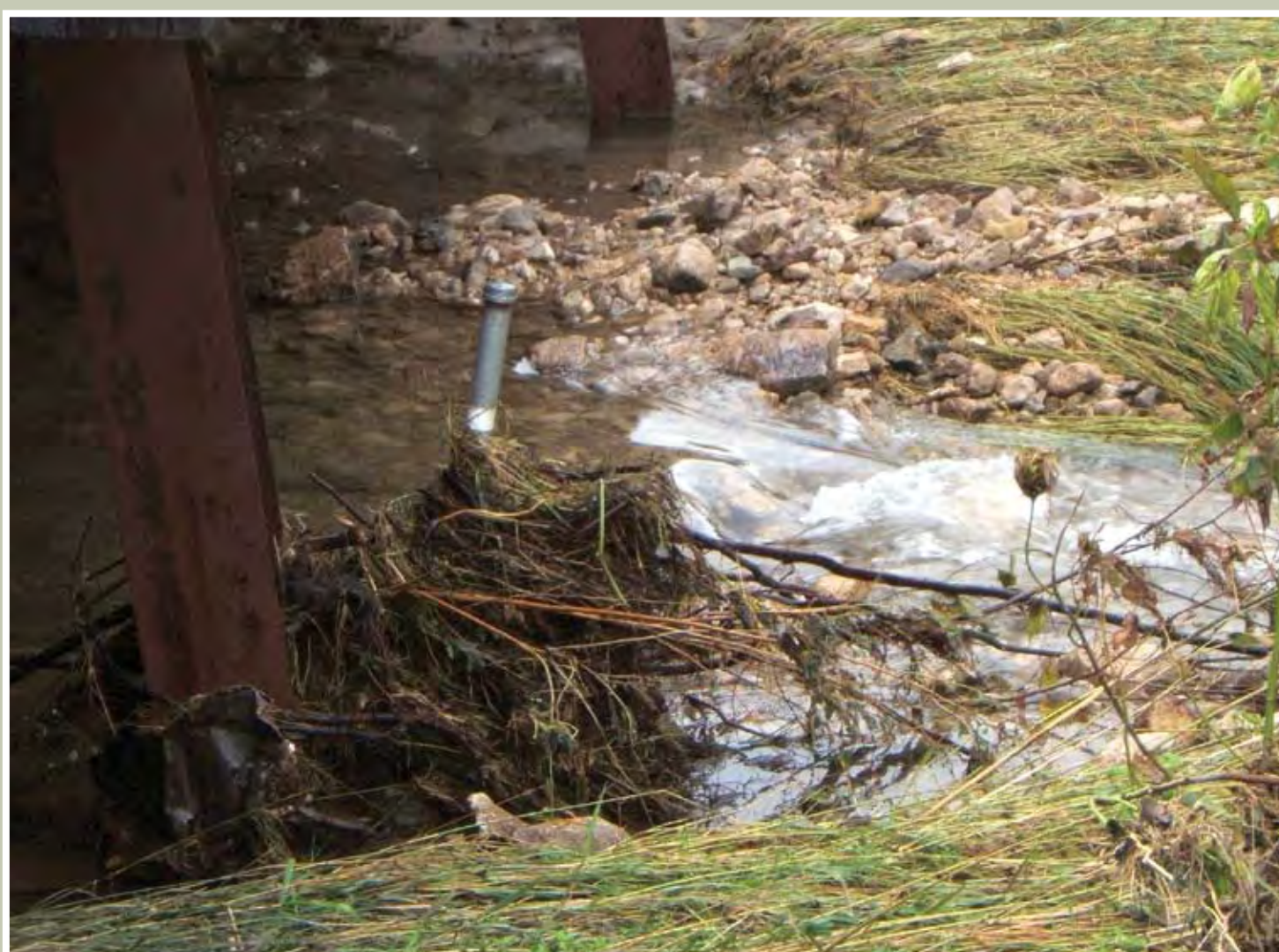
A crest-stage gage damaged by flood debris on Cedar Creek, Minnesota
