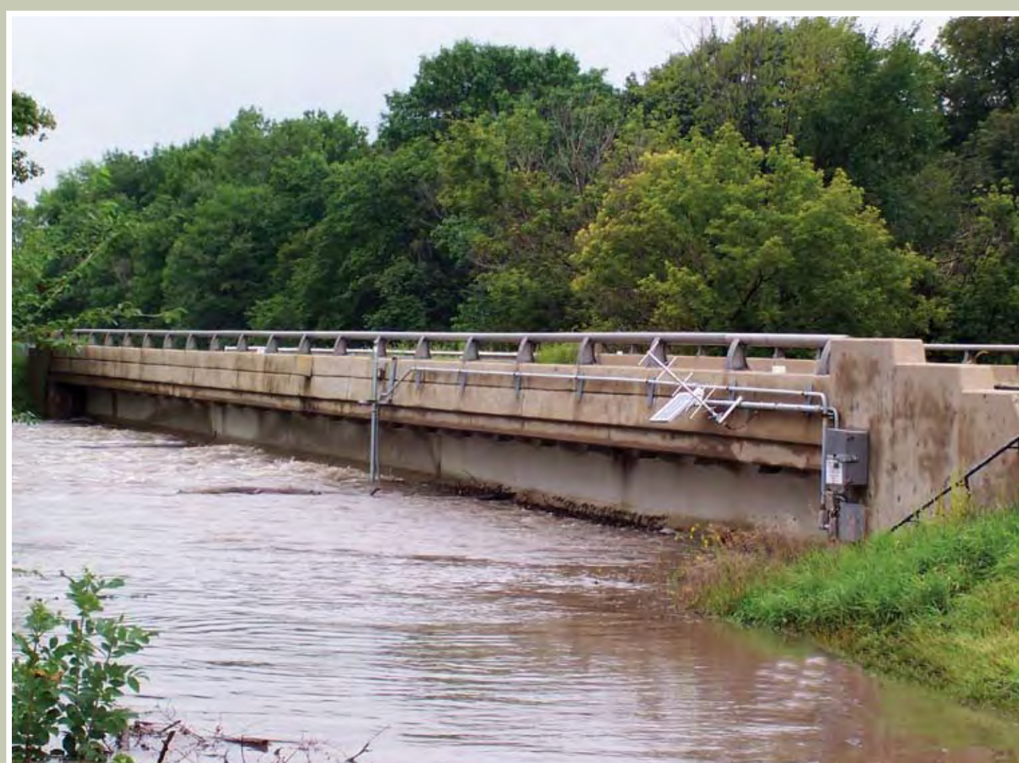
Gaging station on Aux sable Creek, Illinois
