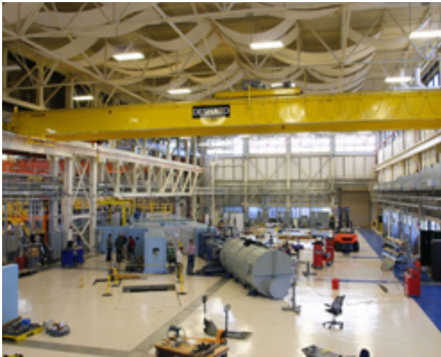
New guide hall with 10 m SANS being placed. Also visible at left are enclosed guides NG-D and NG-C.
