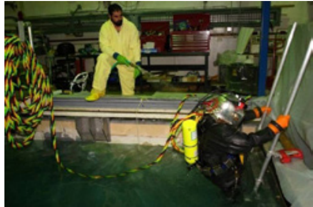
FIGURE 1: Diver (right) exiting the spent fuel storage pool.
