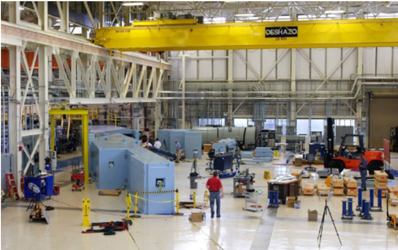
FIGURE 8: Guide installation in G-100. Viewing left to right, the completed NG-D and NG-C guides are seen emerging from end windows of the blue shielding while installation of the as-yet unshielded NG-B guides continues behind.
