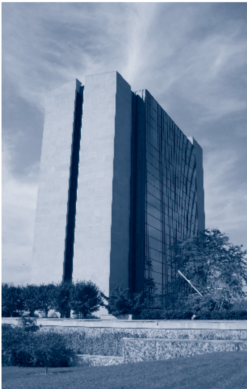
The Lister Hill Center. The NCNR's first home was in its basement.
