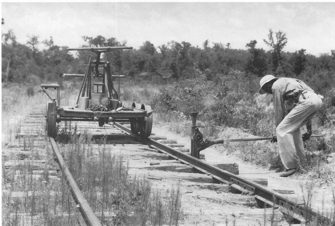
Pulling out the railroad tracks that lead to the closed sawmill, Careyville, Florida, July 1937. (LC-USF34-017727-C) Photo by Dorothea Lange, FSA-OWI Collection, Prints and Photographs Division, Library of Congress
