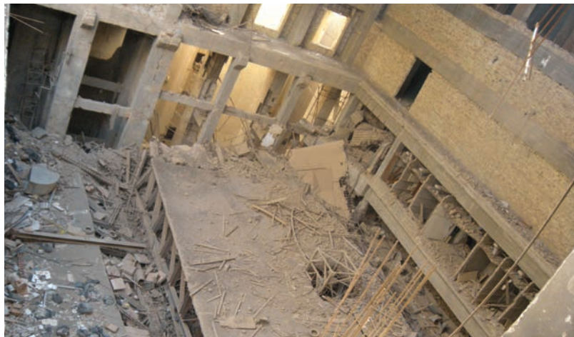
SIGIR’s office building in 2008.
