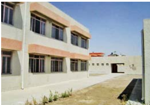
The U.S.-funded Al Khawarizmy Intermediate School in Sadr City. (USACE photo)
