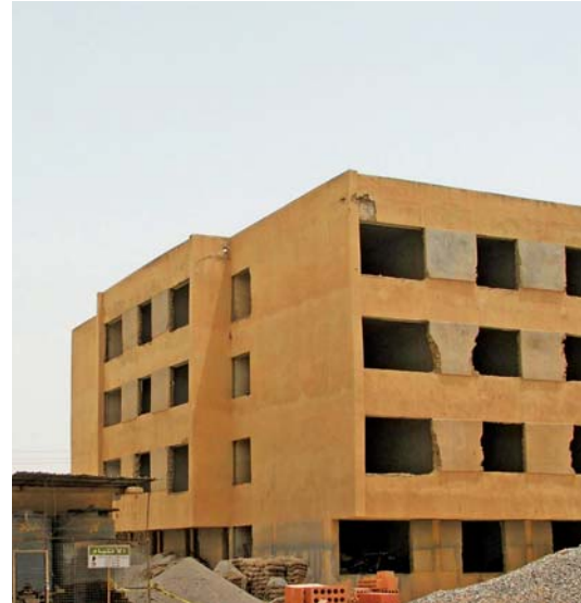
Dormitory at the Hammam Al Alil Regional Training Center.
