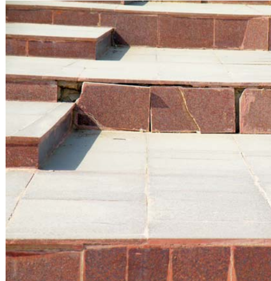
Faulty step work at the Tomb of the Unknown Soldier.
