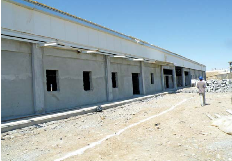
Exterior work at the Rabeaa Point of Entry.
