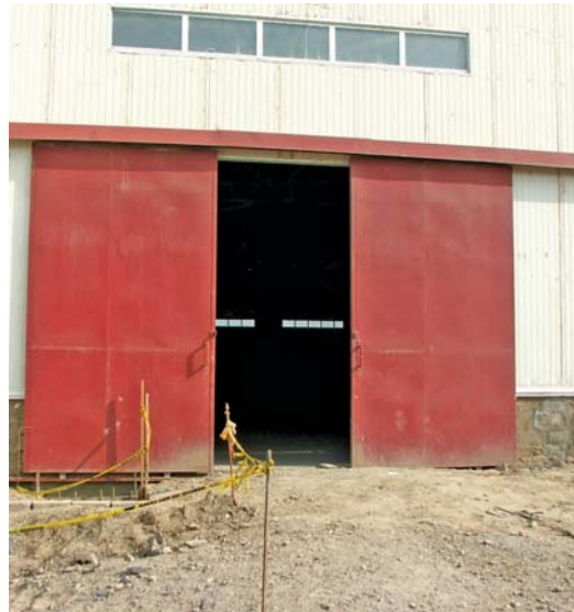
Entry door at the Abu Ghraib Dairy.
