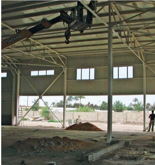
Welding work at the Abu Ghraib Dairy.
