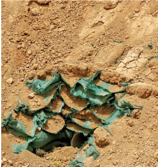
Faulty sandbags at the Hammam Al Alil Division Training Center.
