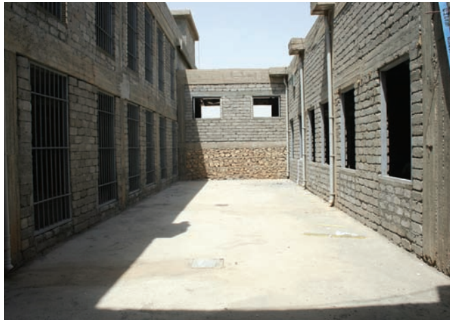
Site Photo 8. Ground-floor installation of security protection bar assemblies.
