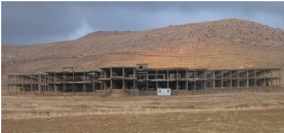
Site Photo 7. The Dahuk Rehabilitation Center at the pre-construction stage for the current contract. (Photo courtesy USACE)
