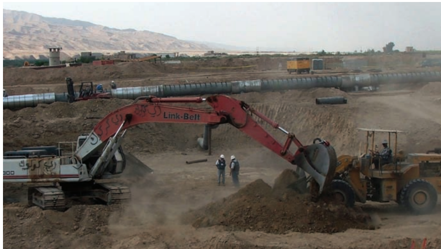
Pipeline construction in northeastern Iraq.
