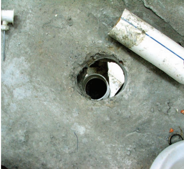
Site Photo 23. Pieces of plumbing pipes in the process of being removed.
