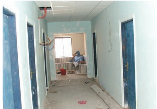
Site Photo 5. Construction in Building B1 (wards, laboratories, and x-ray rooms).
