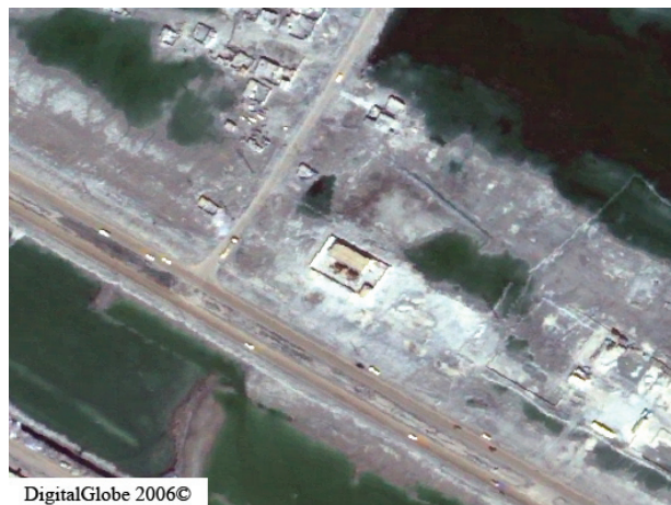
Aerial Image 3. Overview of the Al Hamden electrical substation, which SIGIR personnel visited this quarter.
