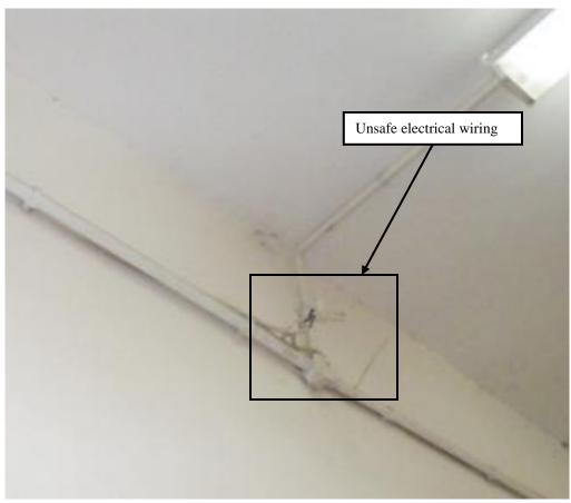
Site Photo 3. Unsafe electrical wiring
