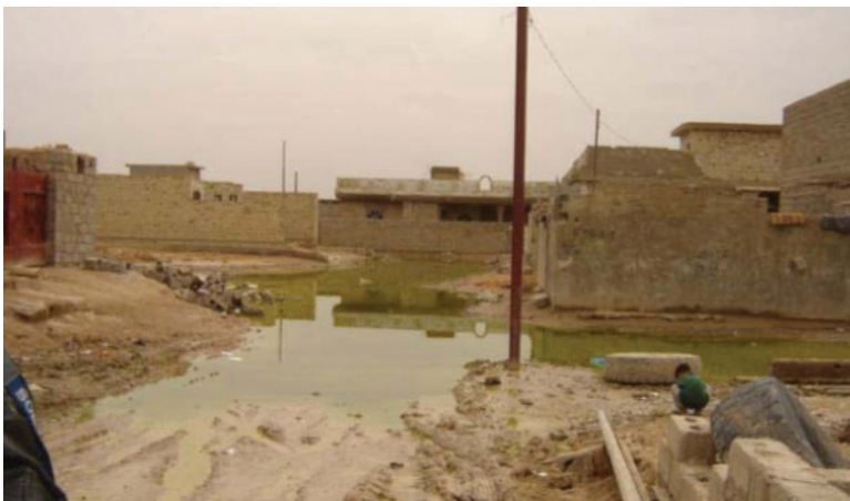
Raw sewage in the streets of Falluja, 2004.
