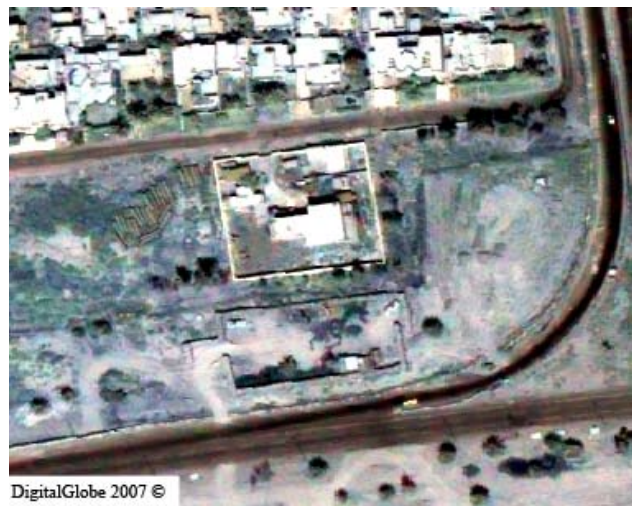
Aerial Image 2. Imagery taken on September 19, 2007, of the Mansour Pump Station, which was assessed in SIGIR PA-07-111.
