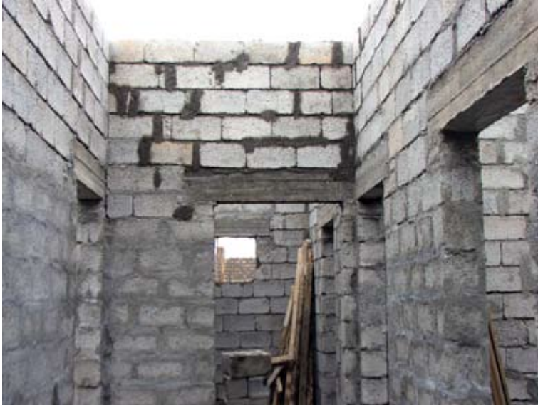
Subcontractor reworked lintels at the Debecha Iraqi Army facility.
