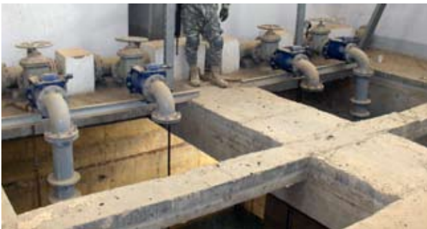
Interior view of the Al Ghazaliyah G-7 building.
