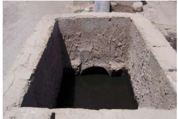
Newly constructed manhole. (Photo courtesy of USACE)
