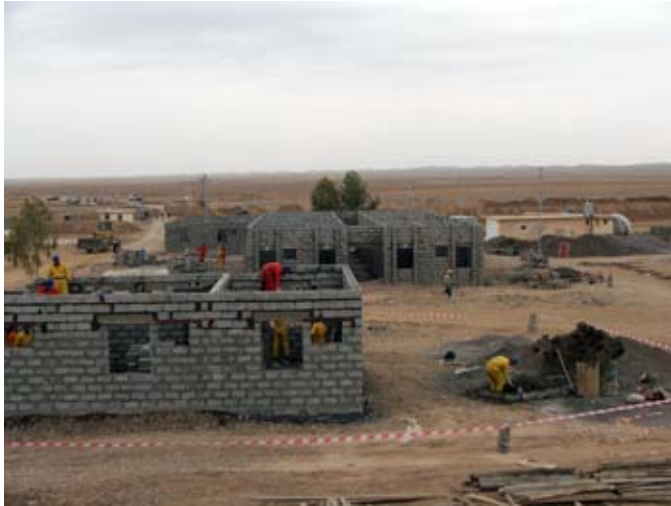
Construction work at the Debecha Iraqi Army facility.
