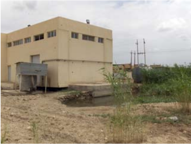
External view of the Al Ghazaliyah G-7 Sewage Lift Station.
