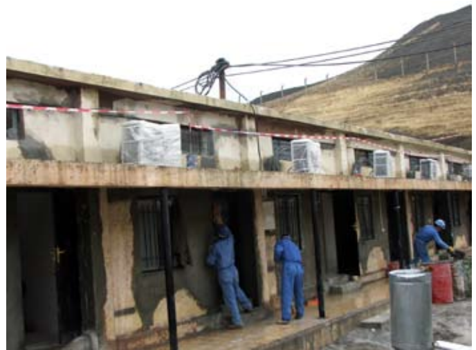
Renovation work at the Diyanah Iraqi Army facility.
