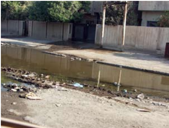
Photo taken November 9, 2007, of the flooded streets in the Al Amerea area of Baghdad outside the Mansour Pump Station.
