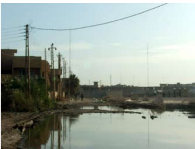
Backed-up sewer water in the Al Ghazaliyah area of Baghdad.
