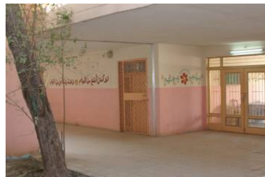
Exterior and interior views of the Al Escanddrone School building after repairs and new paint. (Photos courtesy of USACE)
