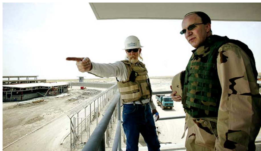
Construction official briefs the Inspector General on the status of construction at the Nassiriya Prison during an on-site inspection in 2008.
