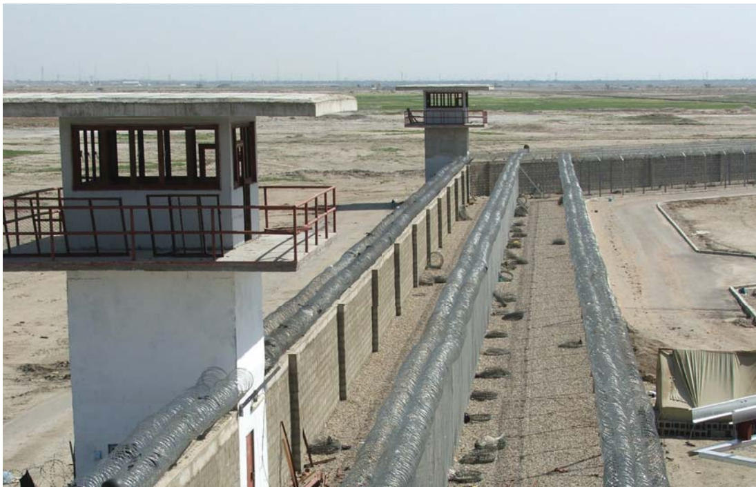
The original contract for construction of Nassiriya Prison was terminated for default after the U.S. government spent $31 million. The project was eventually completed, more than four years later than originally planned, after the expenditure of an additional $37 million.
