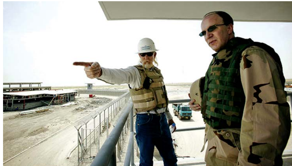
Construction official briefs the Inspector General on the status of construction at the Nassiriya Prison during an on-site inspection in 2008.
