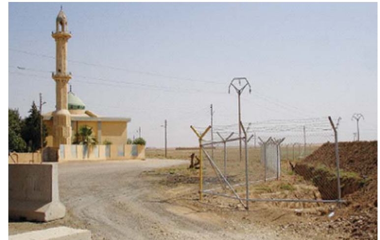
Under the ESF-funded Infrastructure Security Program, the United States supported construction of secured corridors to protect oil pipelines from insurgent attacks. The program contributed to an almost 12-fold increase in northern exports from 2006 to 2008.
